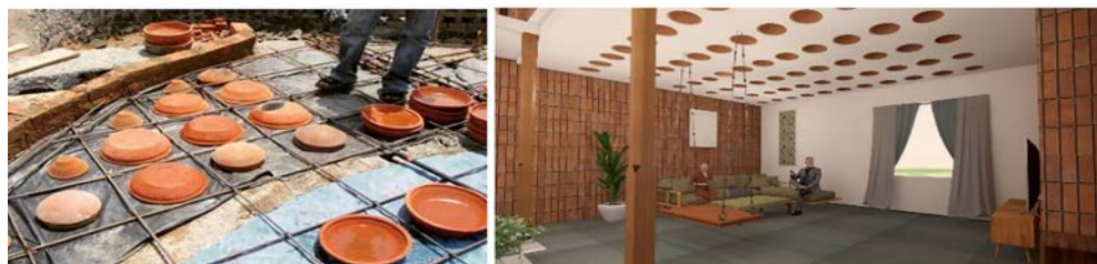
Figure 4. Terracotta Pots Filler Slab (left: construction of the slab, right: finished view of the slab).
