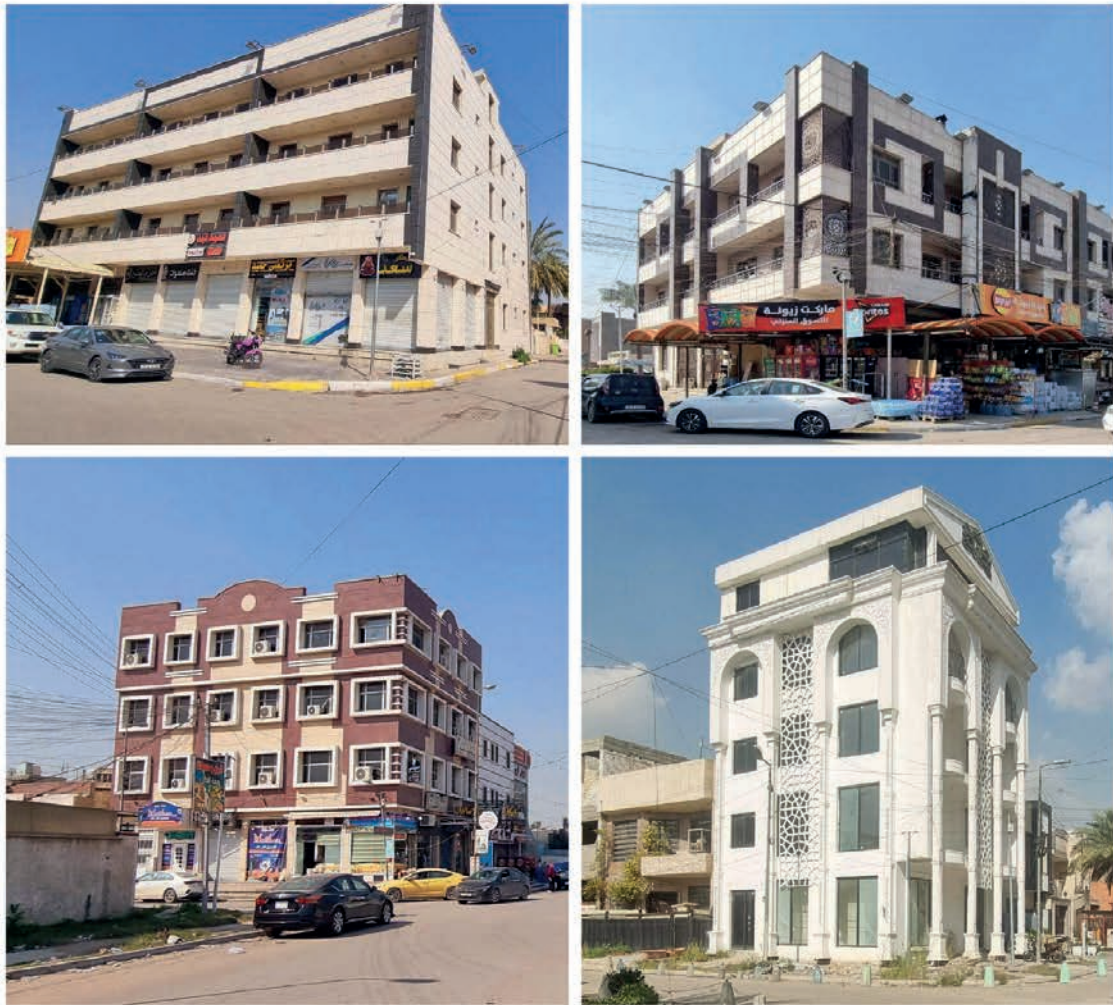
A. Having more than three-floor-height buildings in one residential plot
