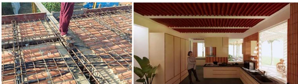
Figure 5. Country Tile Filler Slab (left: construction of the slab, right: finished view of the slab)
