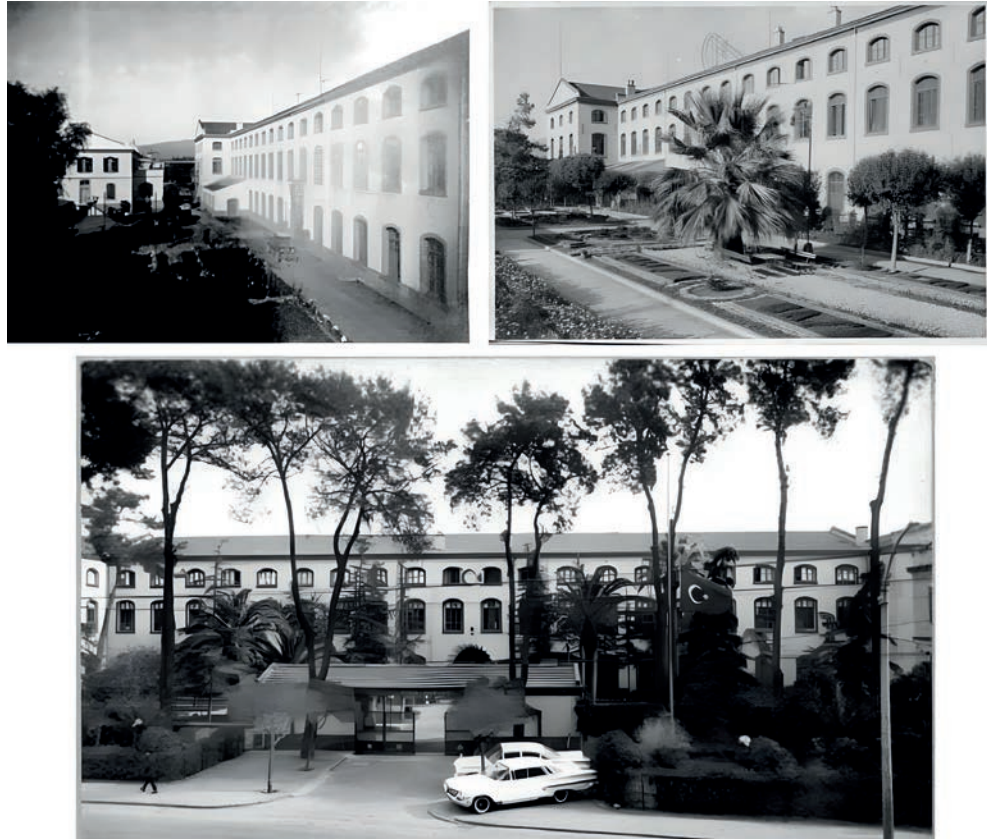
Figure 3. Izmir Tekel Tobacco and Cigarette Factory / Entrance Courtyard. Above: Before and after 1929 (Köksal, 2018, p.69). Below: 1960-1980 (Erol Şaşmaz archive, 2014)
