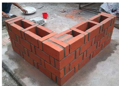
Figure 2. (Left) Arrangement of bricks in Rat trap masonry courses; & (Right) Construction detail.
