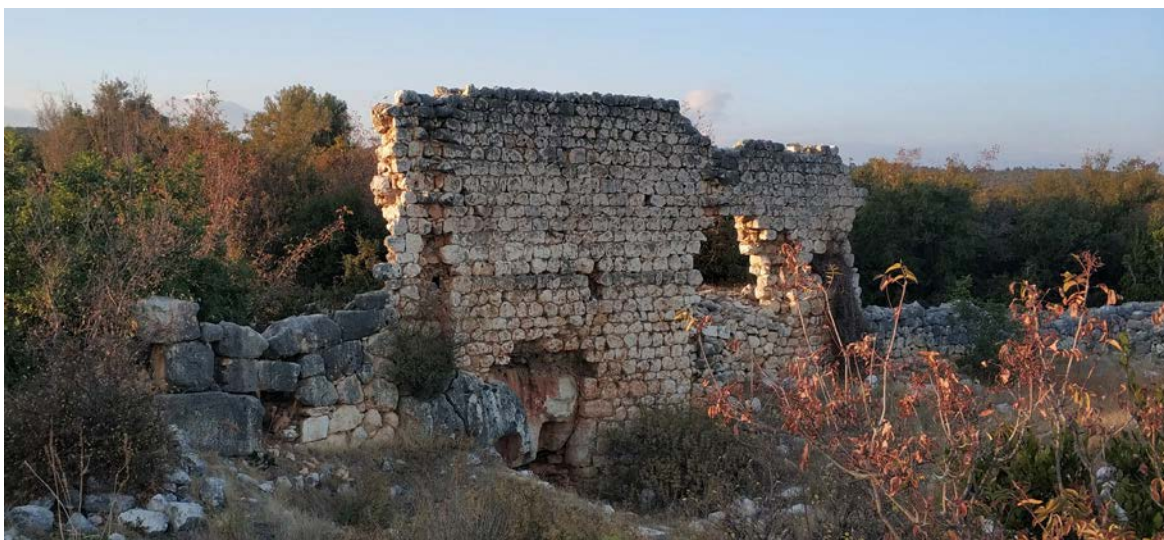
Figure 10. North wall of the market building.
