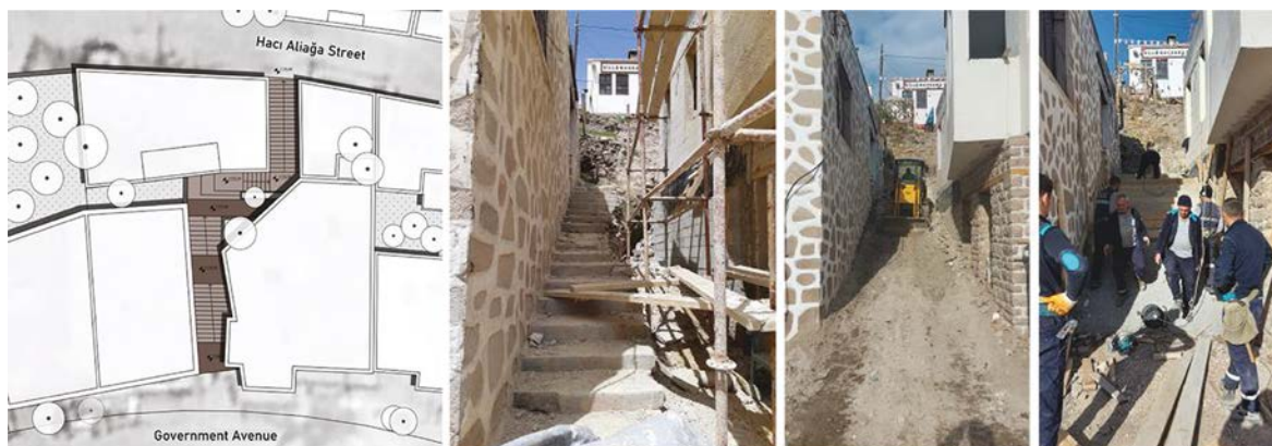
Figure 12. Stepped streets, on site studies.
