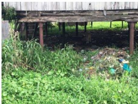
Figure 10. Figure showing round stilts made of steel holding up timber cross beams on which the joists rest. 10
