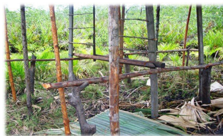
Figure 6. Y-shaped stilt pegs carry the beams, joists and framework for partition wall of the traditional stilt building. 6
