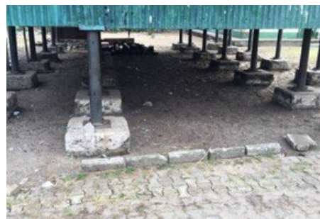
Figure 8. Metal stilts cast in concrete foundation footings. 8
