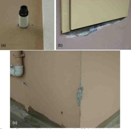
**Figure 3.** Examples of the defects observed at BS-A: (a) delamination at wall-pipe interface, (b) wear off at wall-closet interface, (c) delamination due to impact load.
