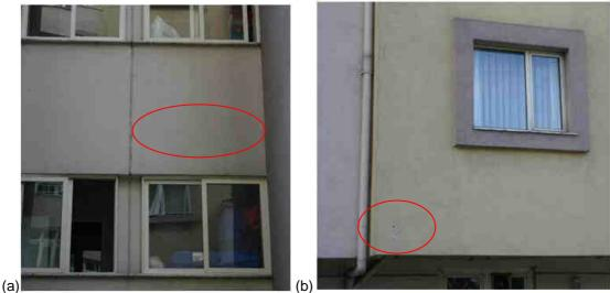
**Figure 5.** Examples from BS-E: (a) crack at floor beam-infill wall interface, (b) drill hole that has not been repaired after the removal of a security camera
