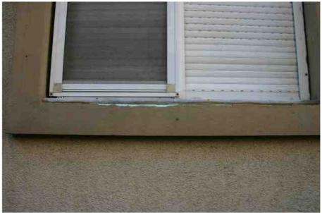
*Figure 7.* Exposure of thermal insulation material to the atmosphere due to wearing off the finish coat at BS-G
