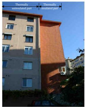
**Figure 1.** An example to the thermal insulation applications carried out during the initial periods of becoming a common practice – the left hand side of the facade is thermally uninsulated and the other part is insulated
