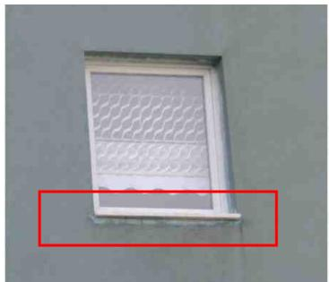
*Figure 4.* Exposure of thermal insulation material due to renewal of window frame and sill at BS-C
