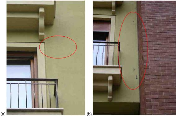
**Figure 6.** Examples from BS-F: (a) isolated crack at window corner, (b) delamination problems that have been occurred due to the impact of falling tiles
