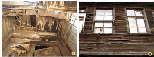
**Figure 3.** Physical deteriorations. a- Deterioration by humidity effects at the ceiling of a timber house in Süleymaniye. b- Deterioration by atmospheric effects on facade of a timber house in Zeyrek.
