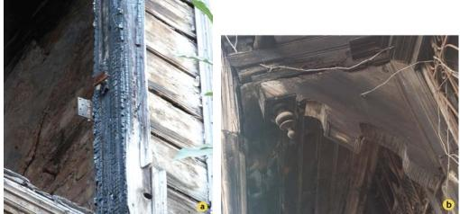
**Figure 4.** Chemical deteriorations. a- A timber house damaged by fire in Süleymaniye. b- A timber house damaged by stove in Zeyrek.
