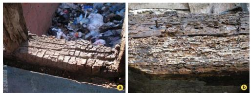
**Figure 5.** Biological deteriorations. a- Timber damaged by wood-destroying fungi. Brown rot fungi are the most destructors of historic timber buildings (Kisternaya and Kozlov, 2009). At the final stages of the attack, wood grows brown in color and breaks apart into cube-shaped pieces. b- Timber damaged by wood-destroying insects. Important pests of timber in historical buildings in this region are beetles belong to the family Anobiidae.
