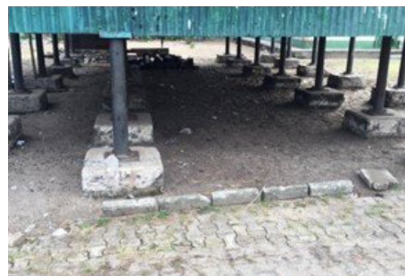
Figure 8. Metal stilts cast in concrete foundation footings. 8
