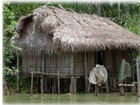
Figure 5. Stems of the palm frond used in construction. 5
