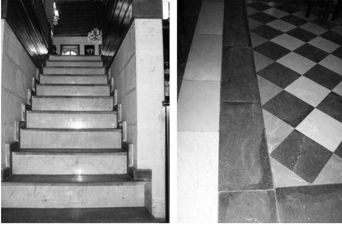
Figure 4. Stairs and floor covering made of Karataş.
