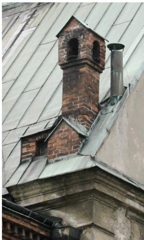
**Figure 9.** Chimney located in the lower corner of the chancel wall gable of the church (Source: Czechowicz, 2018).
