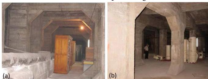
**Figure 5.** Load-bearing members in basement storey for Faculty of Science building (a, b).
