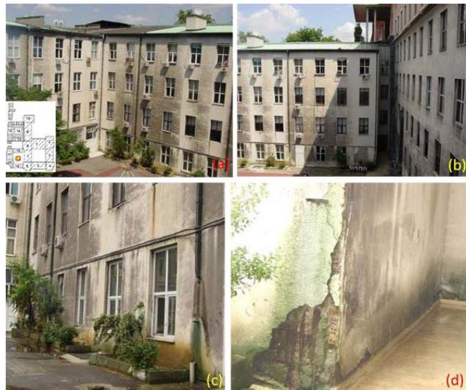
**Figure 4.** Faculty of Aquatic Sciences: (a, b) Inner court, (c) Facade contamination, (d) Corrosion effect in reinforcement.
