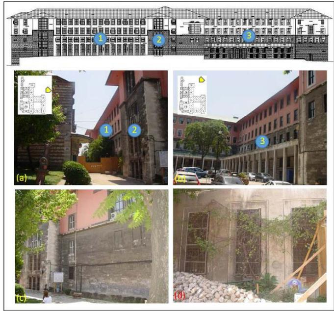
**Figure 2.** Eastern facade: (a) Faculty of Letters, (b) Faculty of Science (c, d) Contamination in facade and window jamb.
