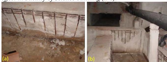
**Figure 7.** RC foundations subject to corrosion effect in Faculty of Letters (a, b).
