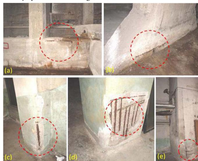
**Figure 6.** RC columns and foundations subject to corrosion effect in Faculty of Science building (a-e).
