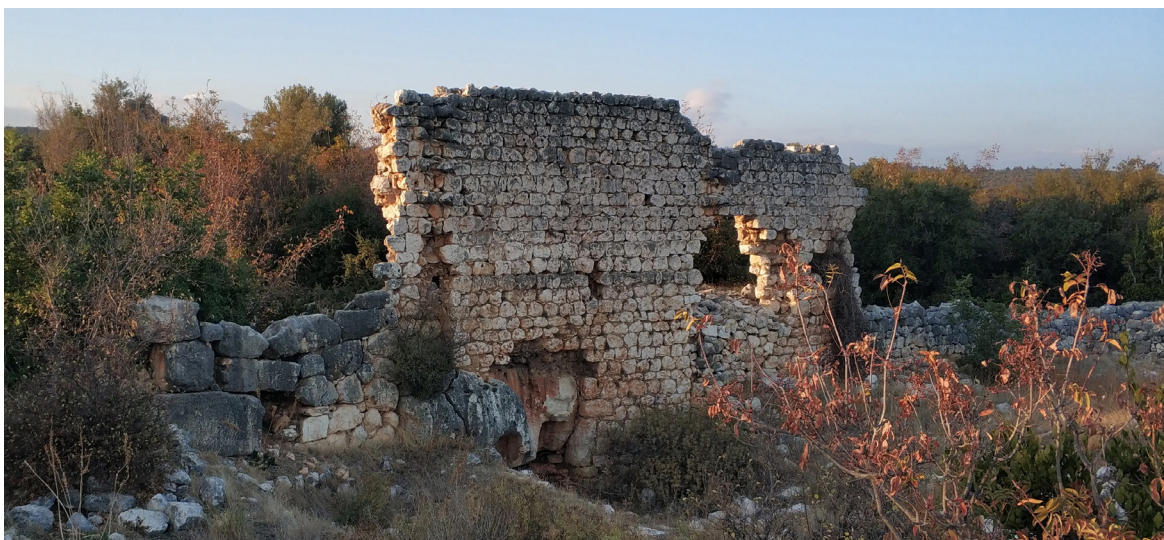
Figure 10. North wall of the market building.
