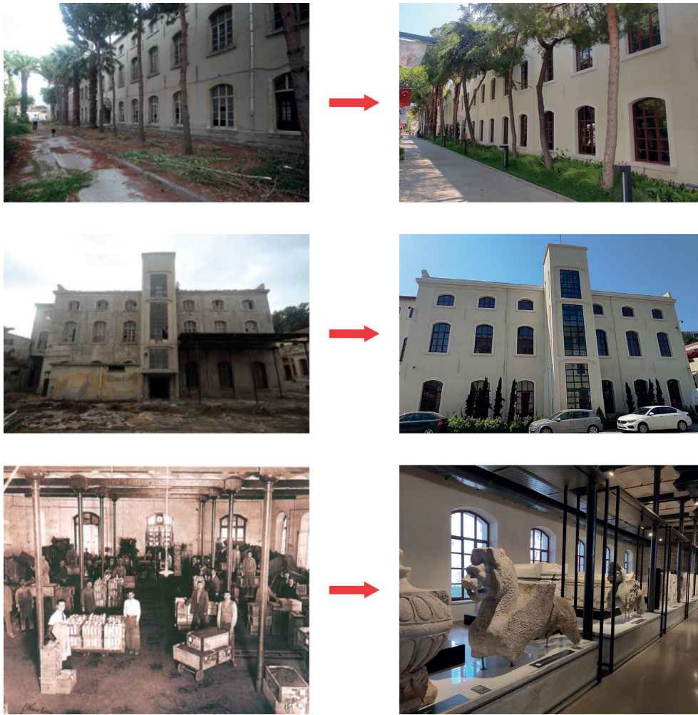
Figure 6. Then and Now: The Production Building / Ethnography Museum. Up & Middle-left: Lift-Es Construction archive in Köksal, 2018; Below-left: Doğruel & Doğruel, 2000, fig.23
