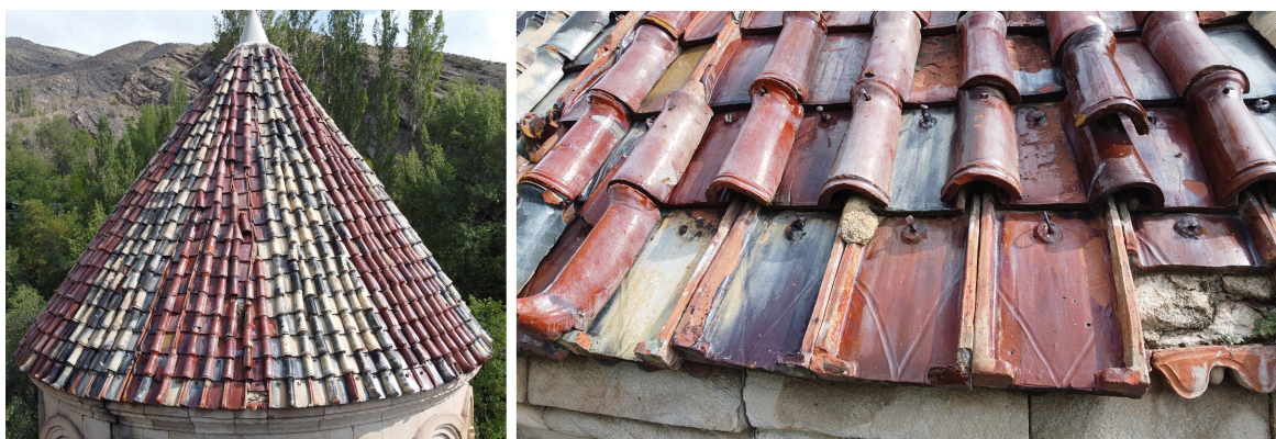
Figure 6. a) Dome cover of Khakhuli's monastic church; b) Detail of the tile cover of the dome (photographs by the authors, 2021).
