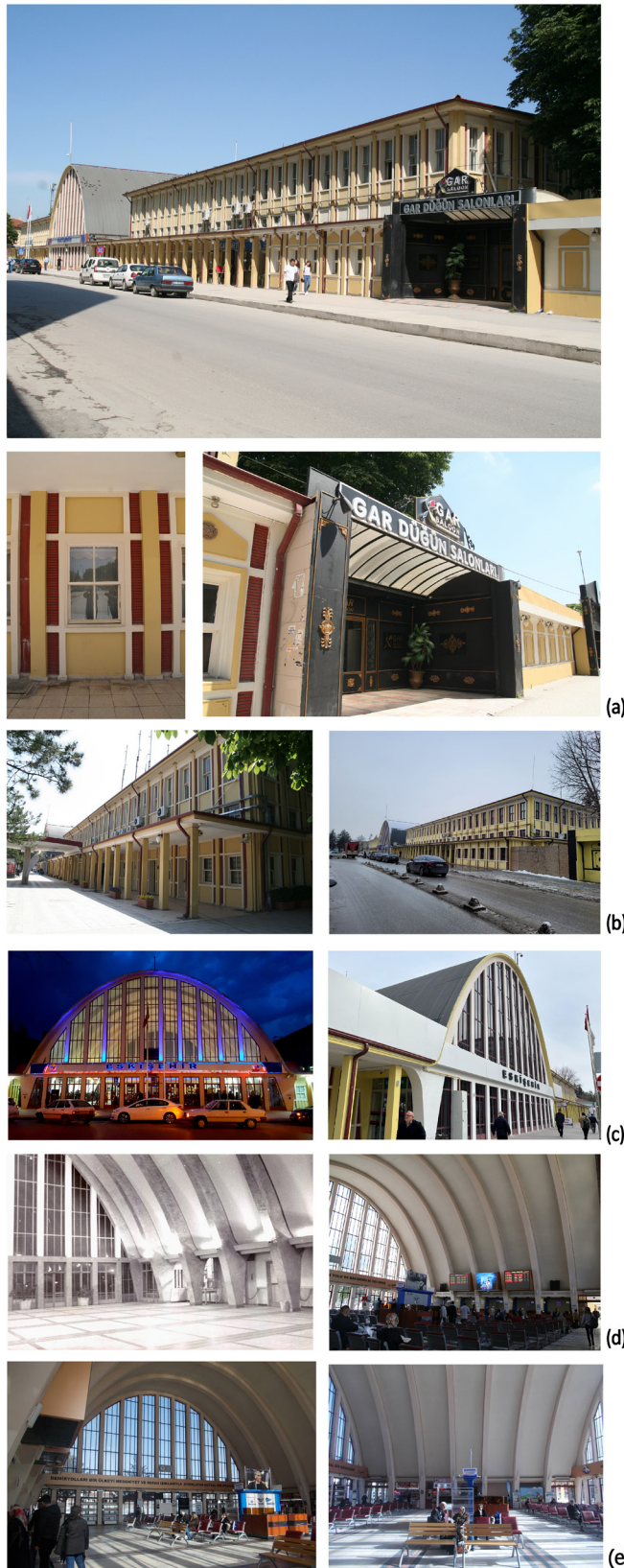
Figure 10. (a) An extension was added to the eastern wing of the building (Binan, 2015); (b) The removal of the addition on the eastern side of the building. (Ulubay, 2022); The eave added to the portico located in the back (railway) facade of the building is incompatible (Binan, 2015); (c) The interior of the passenger hall (1955 and 2016) (Binan, 1955); (d) Eskişehir Railway Station Front Facade (Ulubay, 2018; Polat, 2024); (e) Eskişehir Railway Station The Changes of Interior Design (Tavacı, 2015).
