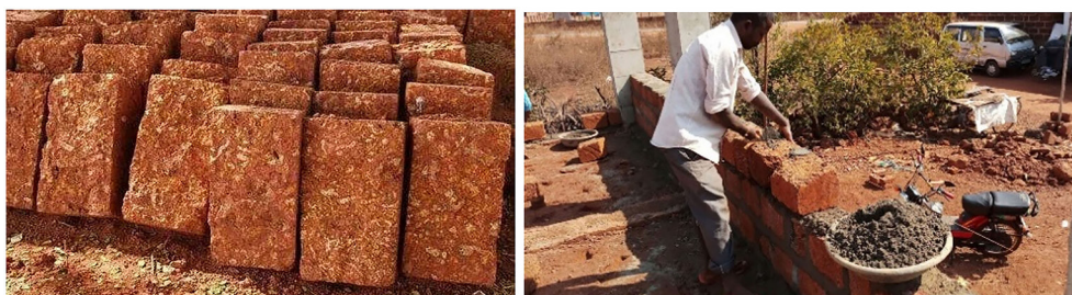
Figure 1. Sample of Laterite stone (Left), Construction of Laterite stone masonry (right).
