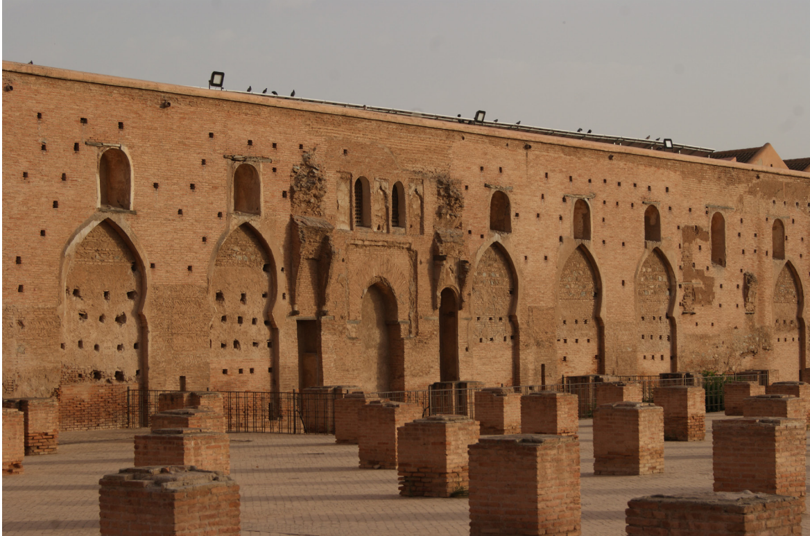
Figure 3. Kutubiyya Mosque (Marrakesh). View of the old qibla with connecting bays between both phases (Author).
