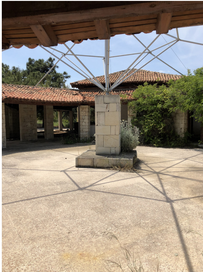
Figure 8. Social facilities designed with yellowish colored local stone and sloped wooden roofs with terracotta tiles differed from the modern design language of the units (photograph by the authors, 2019).
