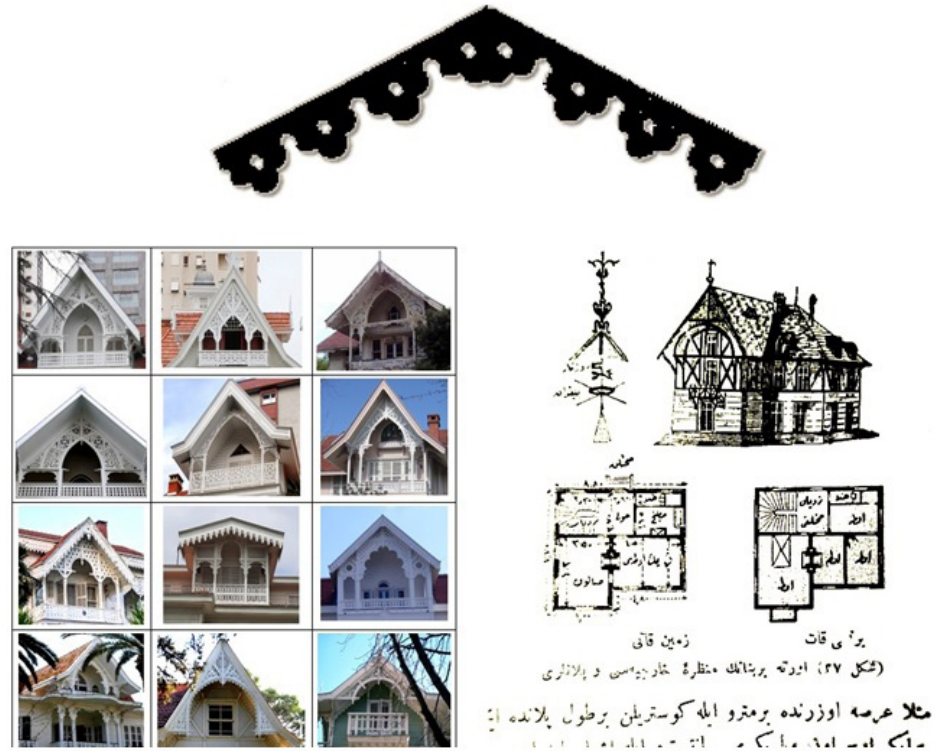
Figure 9. Above: The widely popular type of festoon used on eaves and balcony balustrades (Author). Below Right: The “chalet” type of houses of the era and their layouts, as described by the author Mehmed İzzet in his book (İzzet 1904, Fig 2). Below Left: Kinds of steep gabled roofs. Balconies with Maghribi-Moorish-Orientalist-Mudejar arches and woodworking trim (Author).
