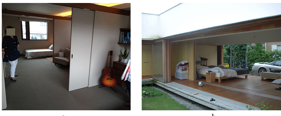
Figure 2. (a) Movable partition. (b) Movable shell in Kairo-no-ye (Cloister House) by Tezuka Architects (Authors, 2019).
