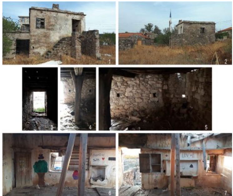
Figure 10. Photos of the house in parcel 1497. 1. West façade, lime plastered surface, exterior stair, slate stone eave, chimney. 2. South façade, partially plastered surface, slate stone eaves. 3. Entrance of the barn. 4. Post, main beam, and secondary beams of the barn. 5. Unplastered wall surface of the barn, niches. 6. Bathing cabinet (yunak), window, shelf, post, and, niche for water jug in the living space. 7. Door, cupboard, match niche, fireplace, post, window in the living space.
