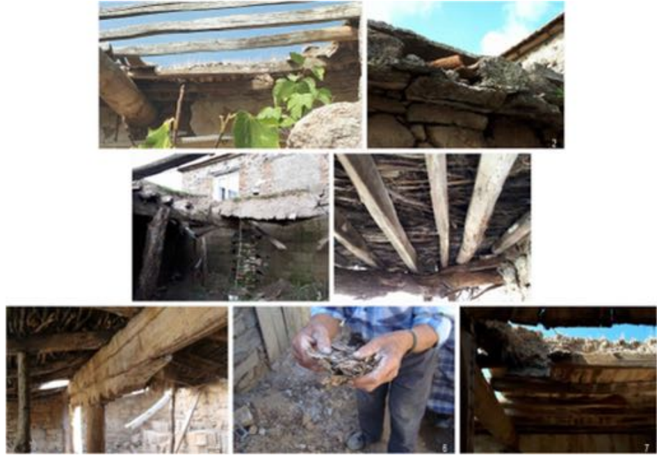
Figure 8. Traditional earthen flat roof elements. 1. Main beam, secondary beams, lath, moss, and earth layers (parcel 1360). 2. Water spout (parcel 1468). 3. Post, main beam, secondary beam, and earth layer (parcel 1468). 4. Secondary beams, branch, bush and moss layers (parcel 1468). 5. Post, bolster, main beam, secondary beams, and sandalwoods as covering layer (parcel 1487). 6. Moss from the roof in the hands of Koşfur (parcel 1487). 7. Main beam, secondary beams, earth layer (parcel 1497).
