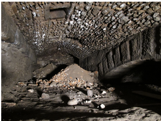
Figure 7. View of the corridor, with the segmental arch of the passage on the right (Author, 2018).
