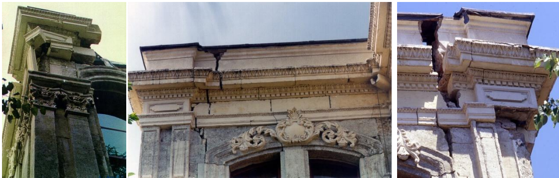
Figure 5. Deep cracks, detachment and material losses at cornice level (increasing in magnitude toward the building corners).
