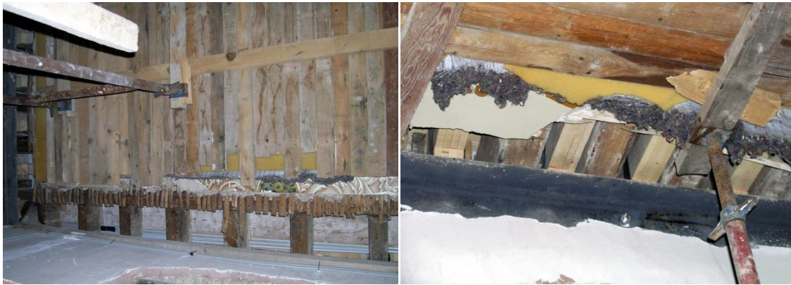
Figure 14. The condition of the intermediate floor structure between the two levels and the transfer of the loads to the load bearing walls from the additional timber beams.
