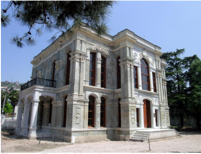
Figure 12. The rebuilding of the parapet wall at roof level with the re-use of the detached fragments.
