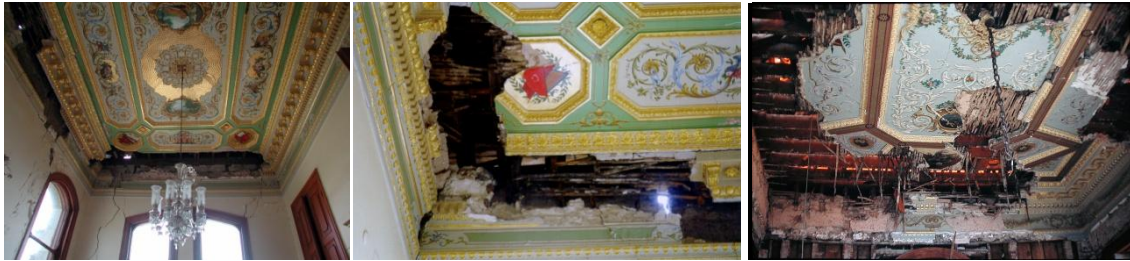
Figure 7. The severe damage on the mouldings and the ceilings.
