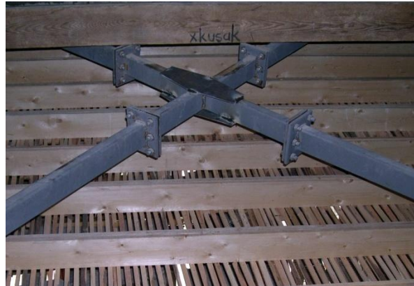
Figure 11. Steel cross-beams were added in the roof space to hinder the outward movement of the main load-bearing walls.
