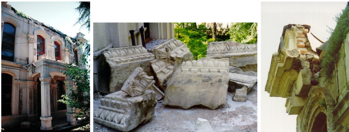
Figure 4. The view of the east façade with collapsed debris of the cornice; these fragments were classified, numbered and then documented in detail with the aim of re-using them in restoration.
