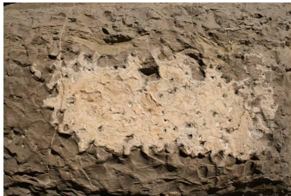
Figure 7. Detachments along the vein of calcite on the façade of Palazzo Medici Riccardi (author's photos).
