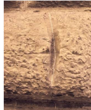
Figure 6. Degradation along the vein of calcite on the façade of Palazzo Strozzi.
