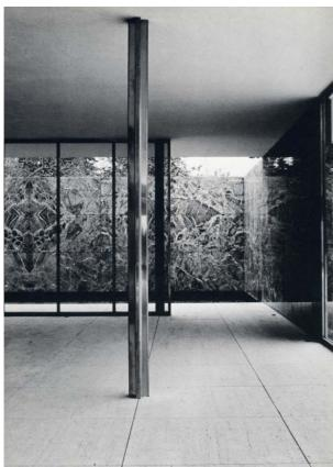
Figure 4. The cross-sectioned stainless-steel columns of the Barcelona Pavilion.
