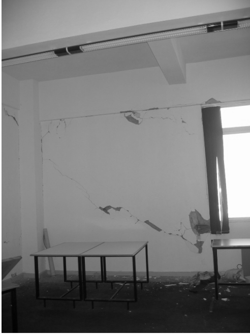
Figure 6 Exterior wall with cracks between structural members and infill material. (Photograph by Şebnem Young).
