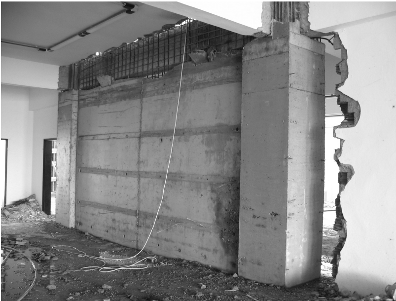
Figure 7 Added shear wall inside Block A. (Source: the Department of Restoration Archive, İYTE)
