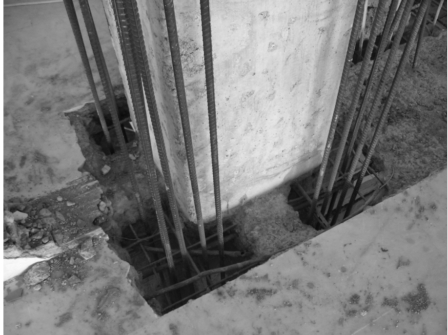
Figure 8 Improved column detail with connecting steel bars. (Source: the Department of Restoration Archive, İYTE).
