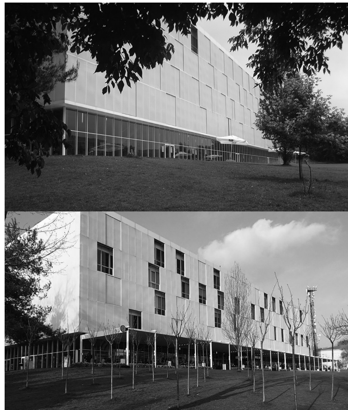
Figure 7. Facade before (above) and after (below) the addition of a canopy (Courtesy of the authors and http://wiki.eanswers.com/tr/%C4%B0stanbul_Teknik_%C3%9Cniversitesi , retrieved 10 February 2016).
