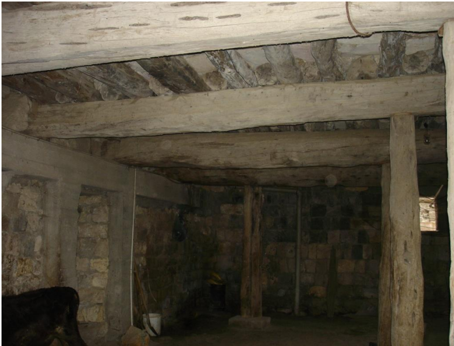
Figure 1. Hezens (central logs) and wooden rafters.
