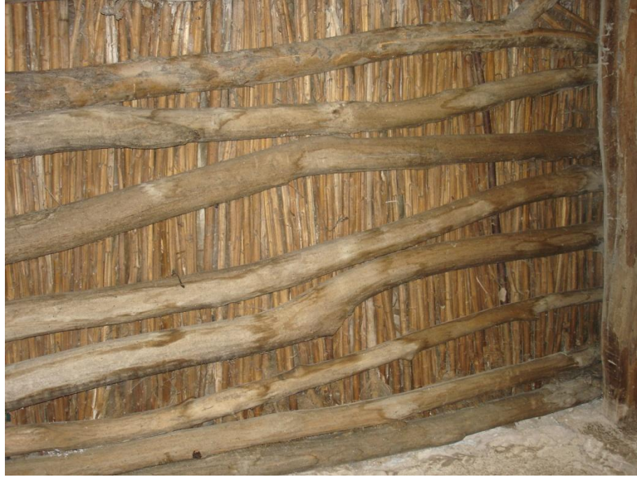
Figure 2. Twigs and reeds placed over the rafters.
