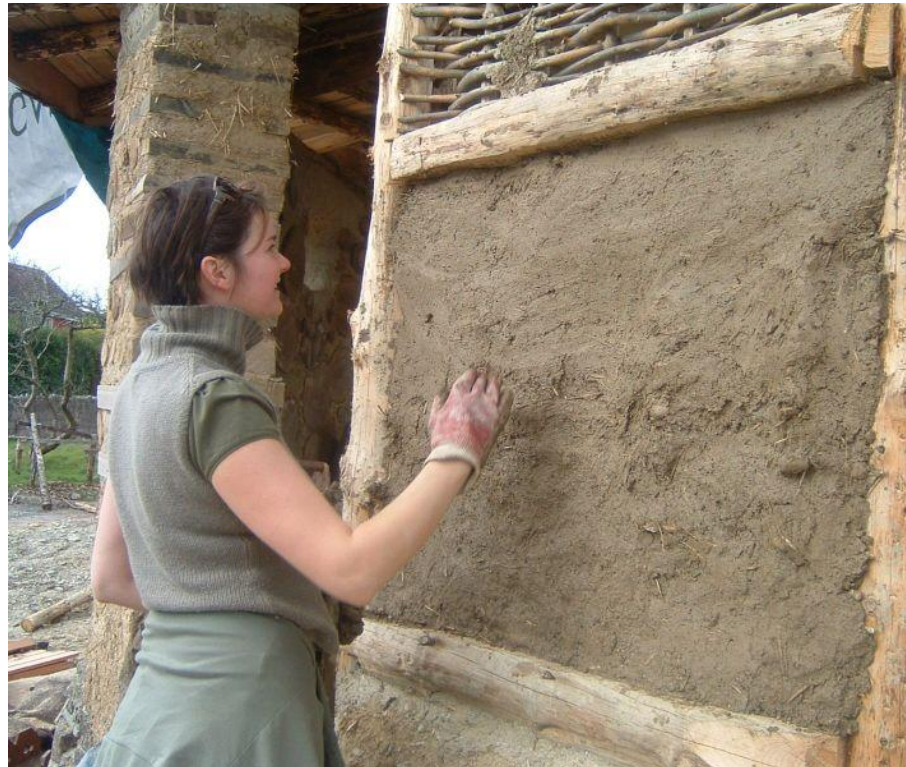
Figure 8. How assorted branches, wicker and mud become a house in Wattle and Daub Technic (Sunshine, 2006).
