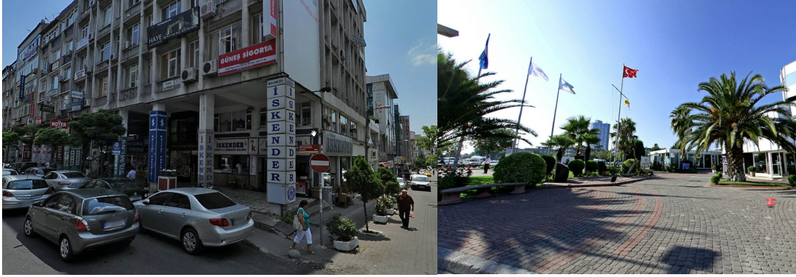
Figure 5. İstanbul Street, sidewalks with colonnade system (left) (source: http://www.yandex.com/ ) and Marina Park in the seaside of Bakırköy (right) (source: http://www.atakoymarina.com.tr/ ).
