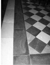
Figure 4. Stairs and floor covering made of Karataş.
