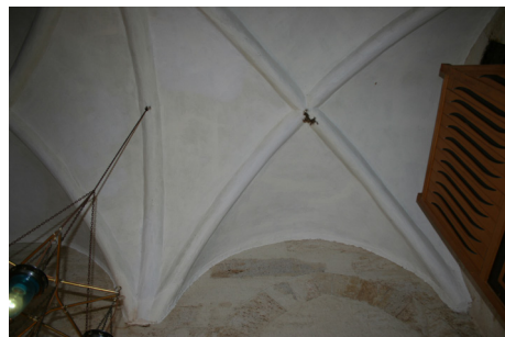
Figure 9. Ribbed cross vault in the building framing the north entrance of the courtyard of Süleymaniye Mosque.
