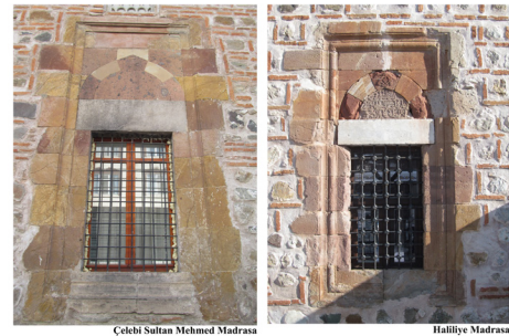
Figure 10. The masonry bond of walls, window mouldings and polychrome stacked window arches of the Çelebi Sultan Mehmed and Haliliye Madrasas.
