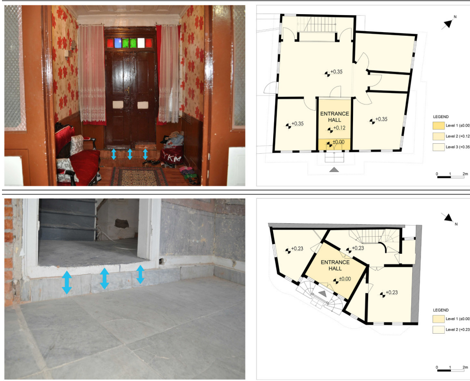
Figure 10. The entrance hole, which is lower than the ground floor level to avoid the dust from being blown into the rooms, Istanbul (Example 1: Photo: Yağcı Ergün, 2012, Drawing: Authors, 2022, Example 2: Photo: Yağcı Ergün, 2015, Drawing: Generated by the authors based on the measurements of Unal, N.).
