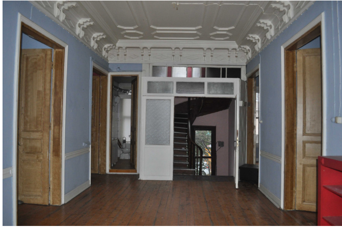
Figure 3. Divisions providing thermal, acoustical and visual isolation from a mansion in Istanbul (Source: Yağcı Ergün, 2015).
