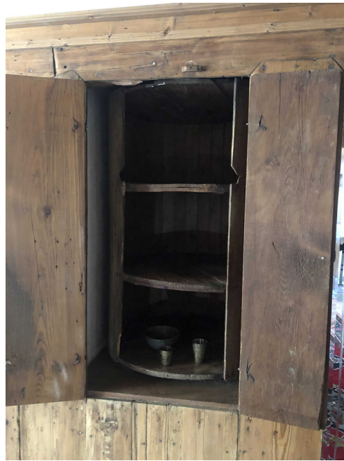
Figure 5. The rotating cabinets used between the Harem and the Selamlık, Safranbolu (Source: Nebioğlu, 2019).
