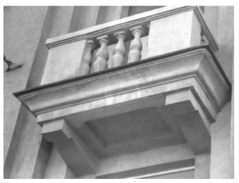
*Figure 2.* Photo of a balcony console for calculations of transverse bending.
