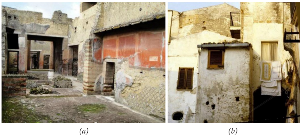
Figure 1. (a) Archetypal surviving (1st century A.D.) exterior stucco rendering on stone-faced concrete walls at Ercolano; (b) an exterior stucco rendering in the Middle East (Bronski, 2010).
