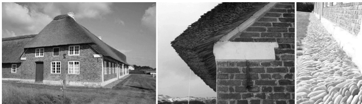
Figure 4. Climate responsive design as seen in Abeline's Farm, showing from left to right: half-hipped roofs reduce wind pressure on the gables, wide eaves protect the building from precipitation and summer sunlight, and pebbles lead precipitation away (Source: Eybye).
